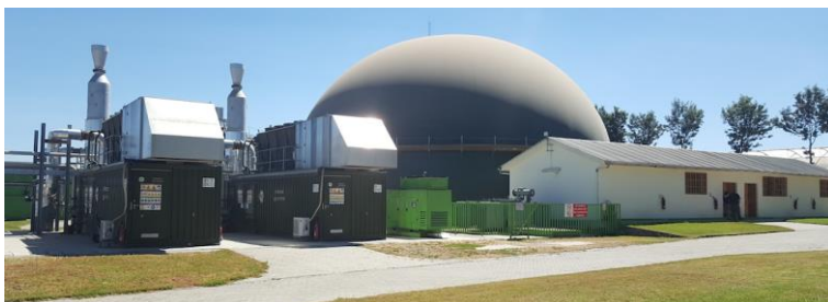
Tropical Power’s grid-connected anaerobic digester in Kenya
